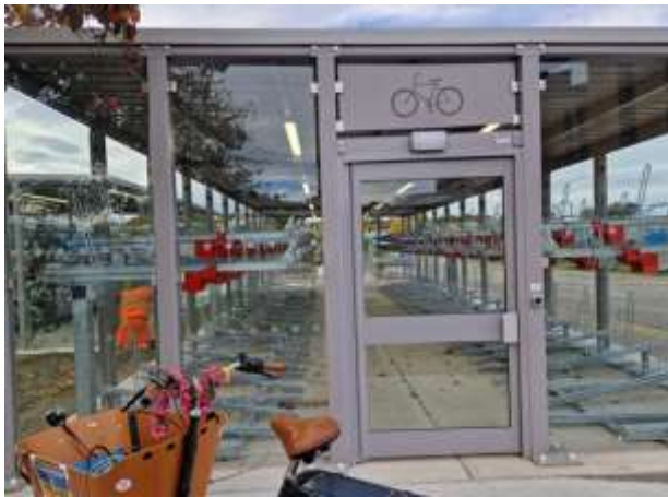
The new secure shelter
